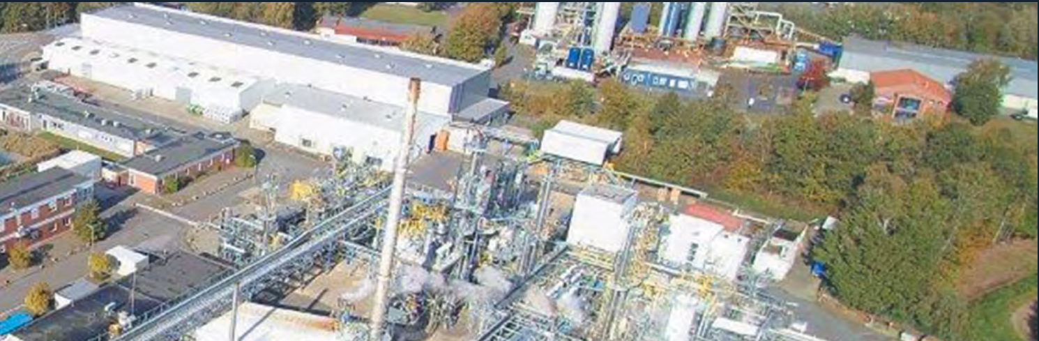
Ibbenbüren, Germany production facility
